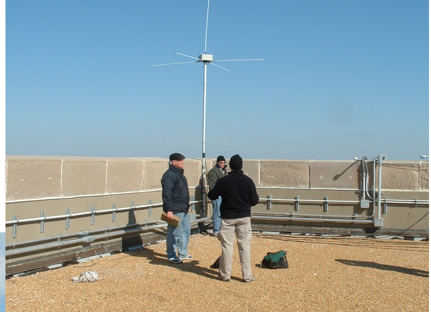
Chesapeake Bay Bridge Tunnel (CBBT)
