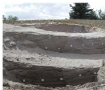
Figure II-14: Sediments from the Borden sand quarry showing an example of preliminary 'stair step' excavations.
