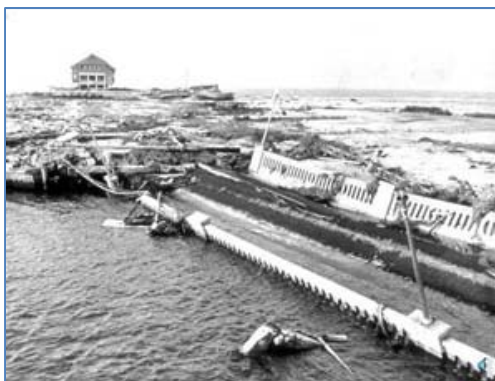
Only a small, sagging portion of the main building of the West Bay Beach Club in Quantuck, Suffolk County, remained after the 1938 "Long Island Express" hurricane.
