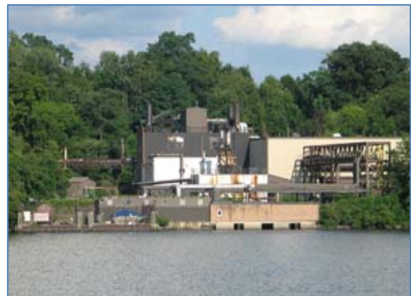
Sea level rise will push the Hudson River salt front upriver, threatening water supplies of several Hudson Valley communities and businesses, including this water intake at the IBM facility in Poughkeepsie, NY.
