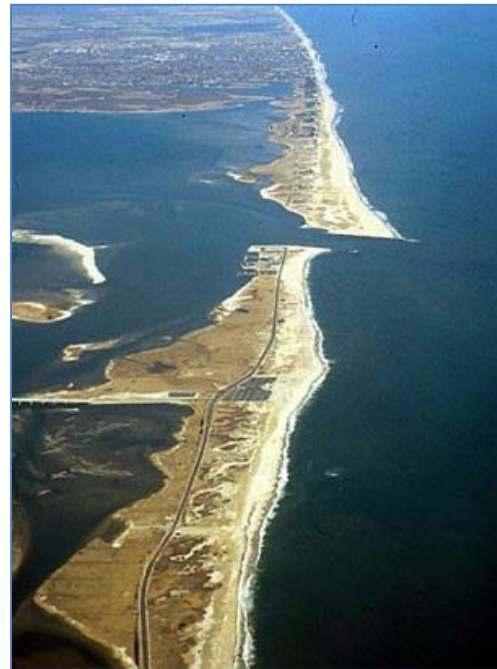
Increased erosion of barrier islands could result in loss of important nesting, foraging and spawning sites. Credit: Jay Tanski
