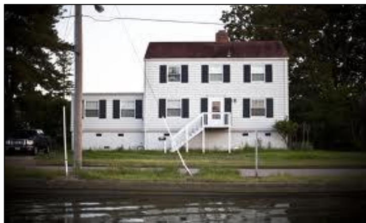
Fig. 8. Flooding in the Lafayette River area.
